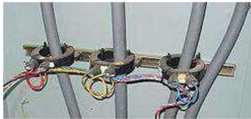
Fig. 15.23 Current transformer
