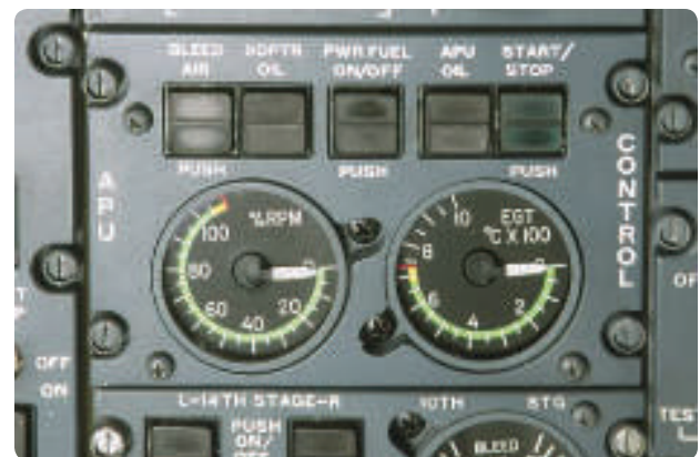
Figure 18-9. A typical APU overhead control/monitoring panel.
