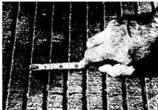
Figure 120 Crosscut runway surfaces drain water rapidly but increase tirewear.
