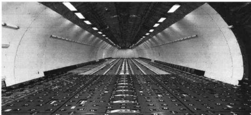
Fig 8.2 Fire protection in a typical cargo compartment. This main deck cargo compartment illustrates two types of fire protection: liners on the sidewalls and smoke detectors running overhead.
