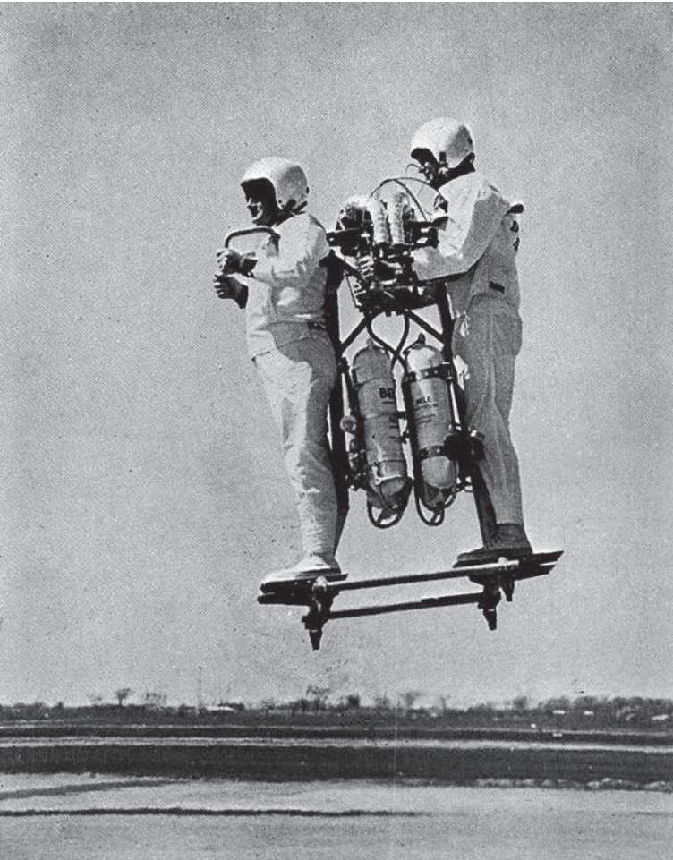
Fig 4D Rocket propulsion (By courtesy of Bell Aerospace Division of Textron Inc, USA) Flying the two-man Pogo from the rear platform is the rocket belt operator; on the front deck is the rocket technician.
