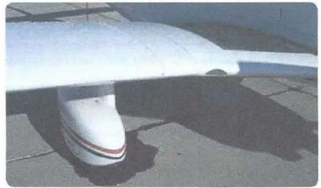
Figure 13-111. The cause of all aircraft brake leaks must be investigated, repaired, and tested before releasing the aircraft for flight.
