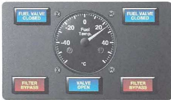
Figure 10-29. A Boeing 737 cockpit fuel panel showing illuminated valve position indicators and fuel filter bypass lights. The fuel temperature in tank No.1 is also indicated.
