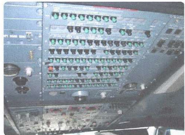
Figure 6-71. Circuit breaker panel.
