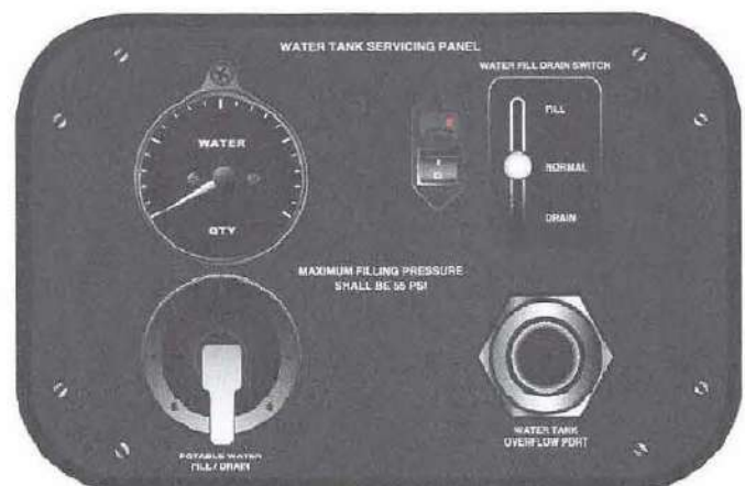
Figure 17-2. A typical water servicing panel on an airliner.
