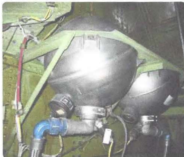
Figure 8-11. Built-in non-portable fire extinguisher containers (HRD bottles) on an airliner.
