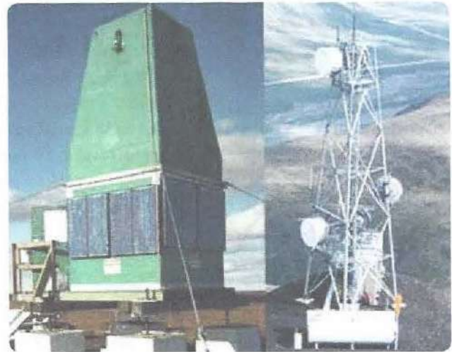
Figure 5-152. Low power requirements allow remote ADS-B stations with only solar or propane support. This is not possible with ground radar due to high power demands which inhibit remote area radar coverage for air traffic purposes.
