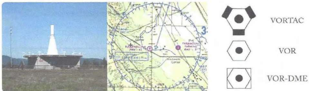
Figure 5-112. A VOR ground station.
