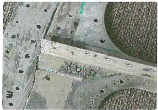
Figure 4-7. Concentration cell corrosion.
