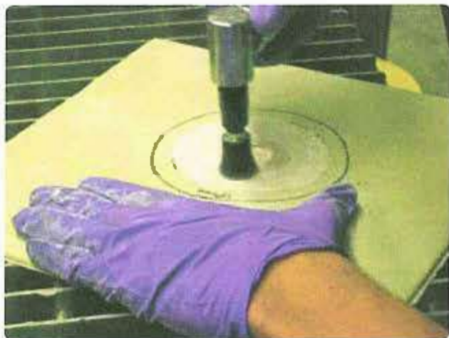
Figure 3-60. Taper sanding of repair area.
