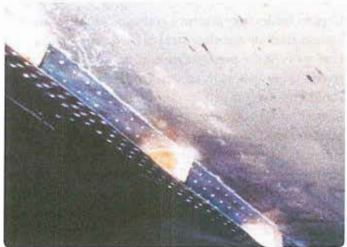
Figure 4-25. Opening of a corroded lap joint for repair.
