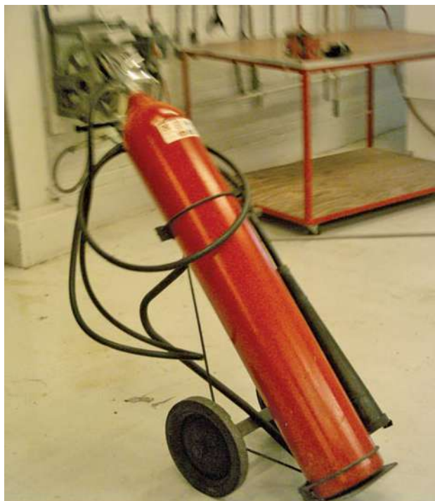
Figure 11-4. Carbon dioxide fire extinguisher.
