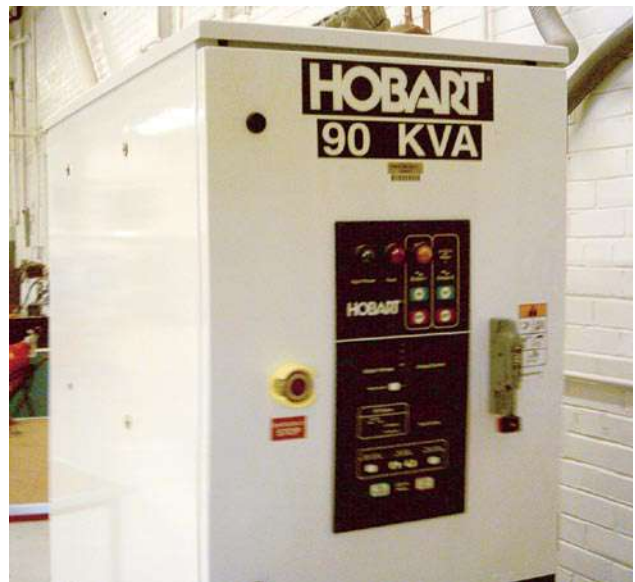
Figure 11-28. A stationary electrical power unit.
