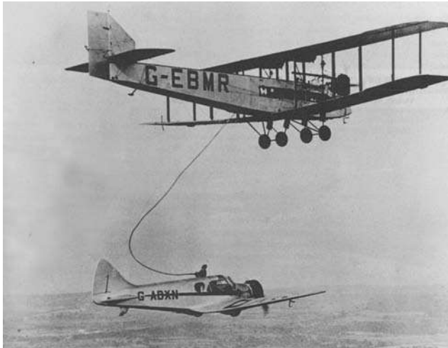
Figure 3.1 Handley Page W 10 tanker refuelling Sir Alan Cobham's Airspeed Courier in October 1934. S/Ldr W. Helmore had the draughty task of handling the fuel hose (Courtesy of Flight Refuelling Ltd/Cobham)
