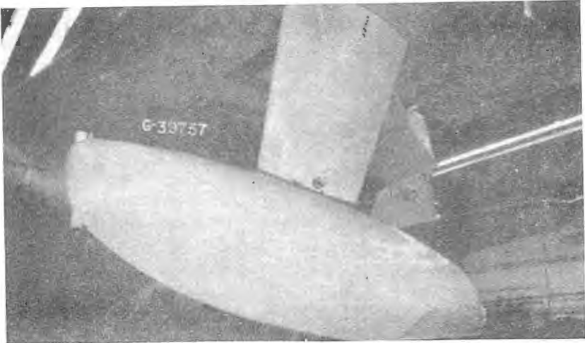
FIGURE 42. Wing-tip Float and Bracing: Aluminum-alloy Sheet and Tubing
